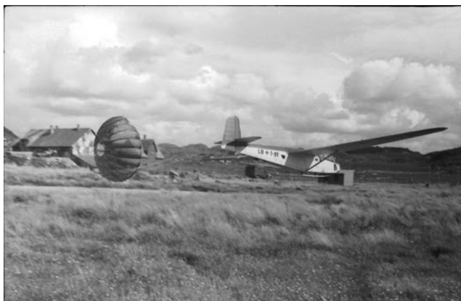
Figure 1 DFS 230 rounding out after an 80 degree parachute retarded approach.
